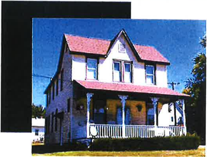
612 Front St. Trim & Gutters
