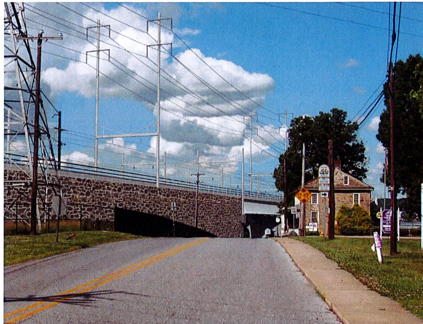
Photo 79: Rendering showing the proposed retaining wall to be constructed in front of Rodgers Tavern, with a possible aesthetic design solution.
