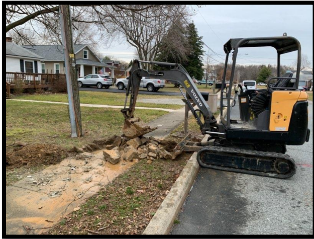
The mini excavator removing a section of sidewalk to prepare for a water repair.
